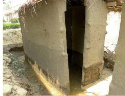
NEM plastered versus traditional mud plaster tested for water resistance. Bitumin NEM to the left.JPG
