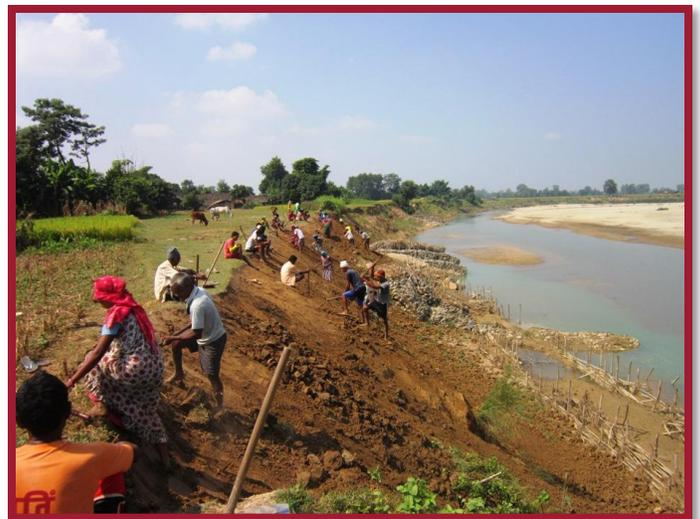
Flood risk is reduced by bio-engineered mitigation works, such as building bamboo spurs and locally selected plants to hold the riverbank in place. Photo: Nabin Lamichhane/Mercy Corps
